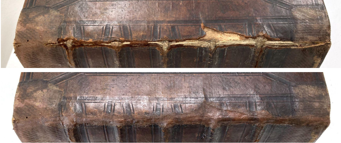
Fig. 13. Broken joint before (top) and after (bottom) treatment, by Kristin. The repair was made to match the leather in colour and gloss.
